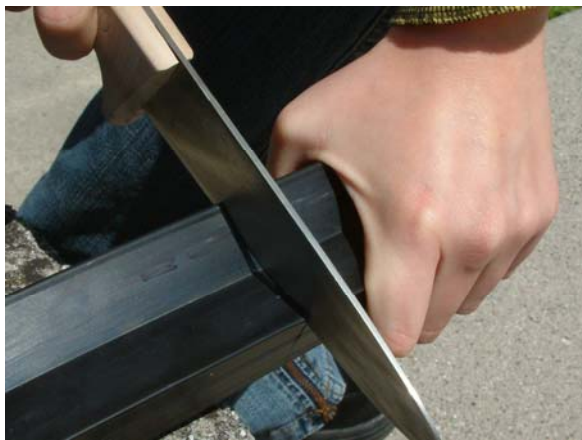
Cutting to length of a bull wheel liner
